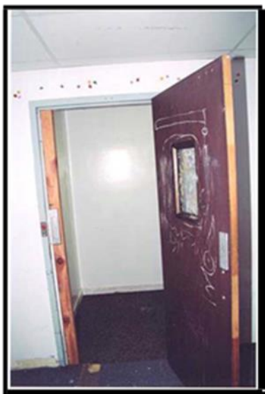
Original locked seclusion room.
