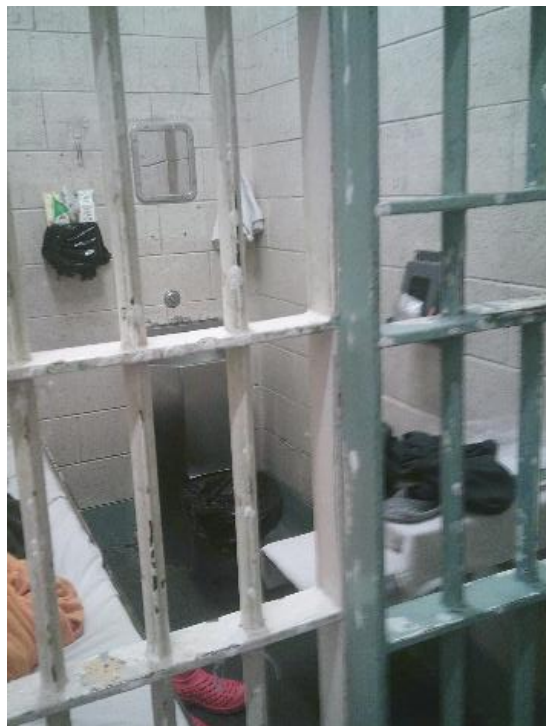
Photo: Isolation cell, with little room to stand, and with bars that have been used by suicidal incarcerated people as tie-off points
