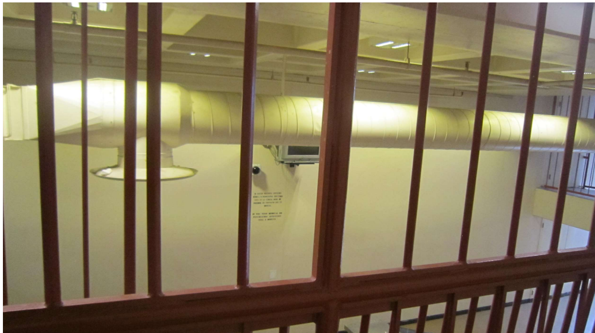
View of the Dayroom Television from Outside of a Cell on the Second Tier
